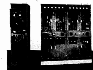
Western Electric 250 Watt equipment at Station WPRO. Left: 220A Volume Indicator Panel and 59A Amplifier. Right: 12A Transmitter and 71A Amplifier.
